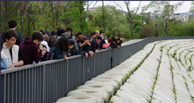
Students look over a new barrier at the flood site
